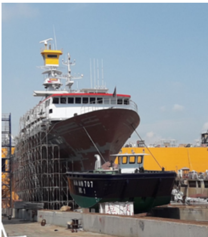
Fair Well's newest vessel, Vanuatu-flagged Win Win 707, in the final stages of construction at Jong Shyn Shipyard, Kaohsiung, May 2019
